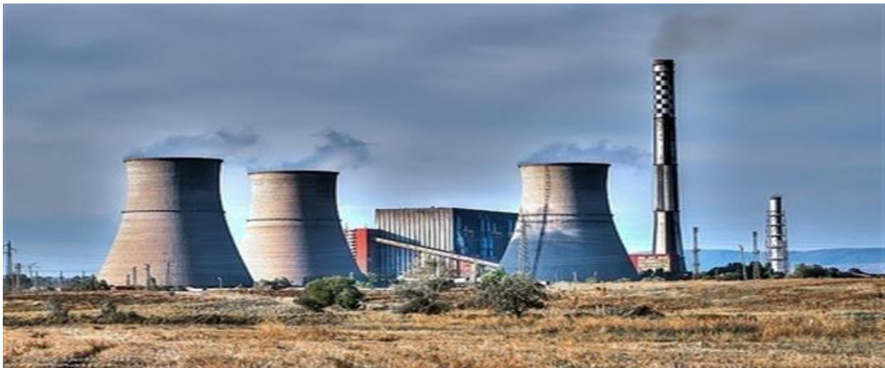
Picture of Munyati Power Station
