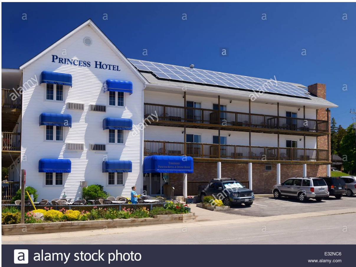
Figure 2.3: Solar panels on the roof top of Princess Hotel
